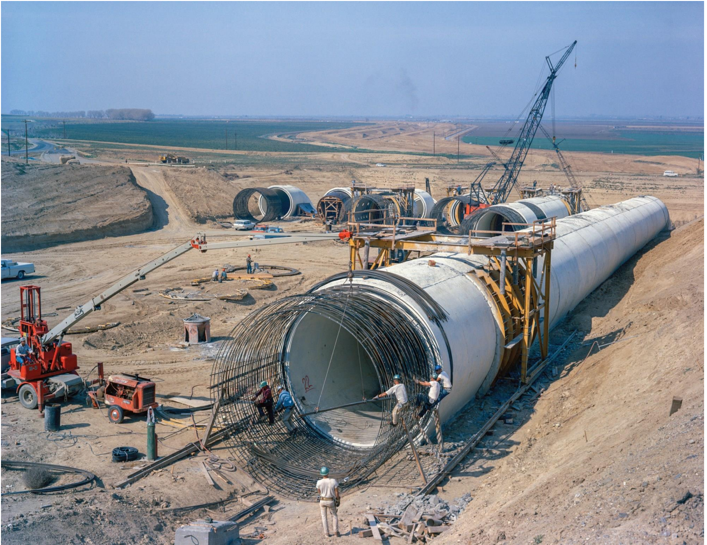
Workers assemble the rebar for the construction of a discharge line at the Dos Amigos Pumping Plant site, built on the California Aqueduct-San Luis Canal in Merced County, California. The State Water Project facility, which was completed in 1966, would lift waters over 100 feet from the aqueduct as it continues its southern path for the SWP. Photo taken March 12, 1965 Bob Dunn/California Department of Water Resources
