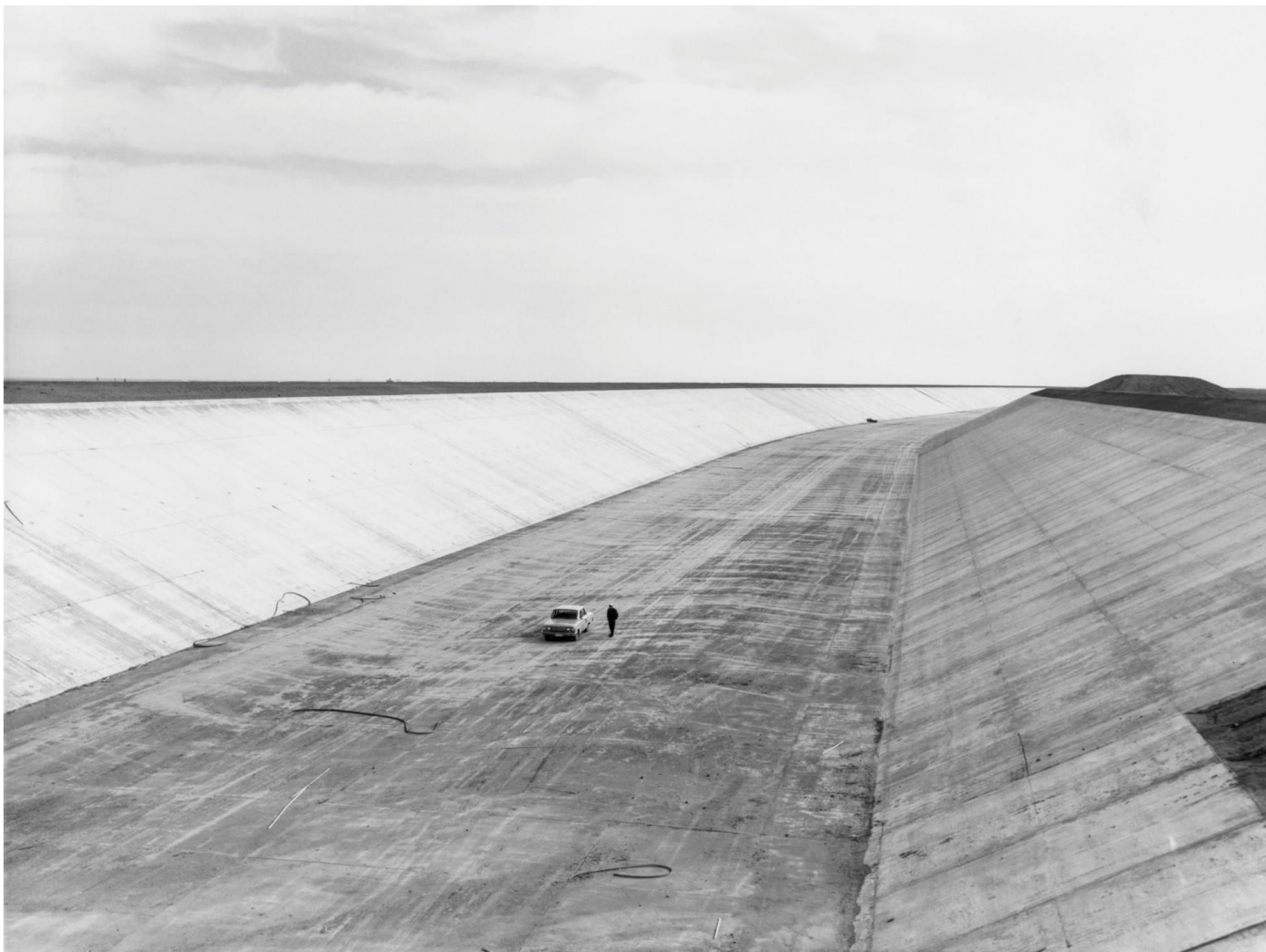
A vehicle is dwarfed by the size of this completed section of the San Luis Canal/California Aqueduct, which is part of the Central Valley Project and California State Water Project in Merced County, California. Photo taken Feb. 17, 1966. J.C. Dahilig/Bureau of Reclamation
