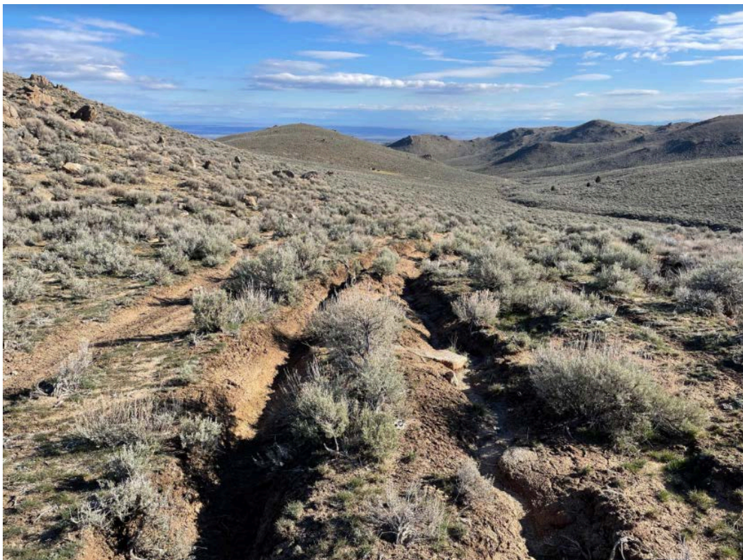
Significant gullying farther downslope along trail GVX1288 in Hogpen Gulch
