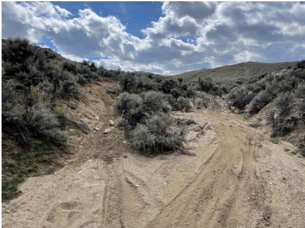
The bottom section of Route ID: 37GV4165.100 is mostly sand wash but steeper sections are experiencing erosion from dirt bikes and could benefit from trail stabilization work.
