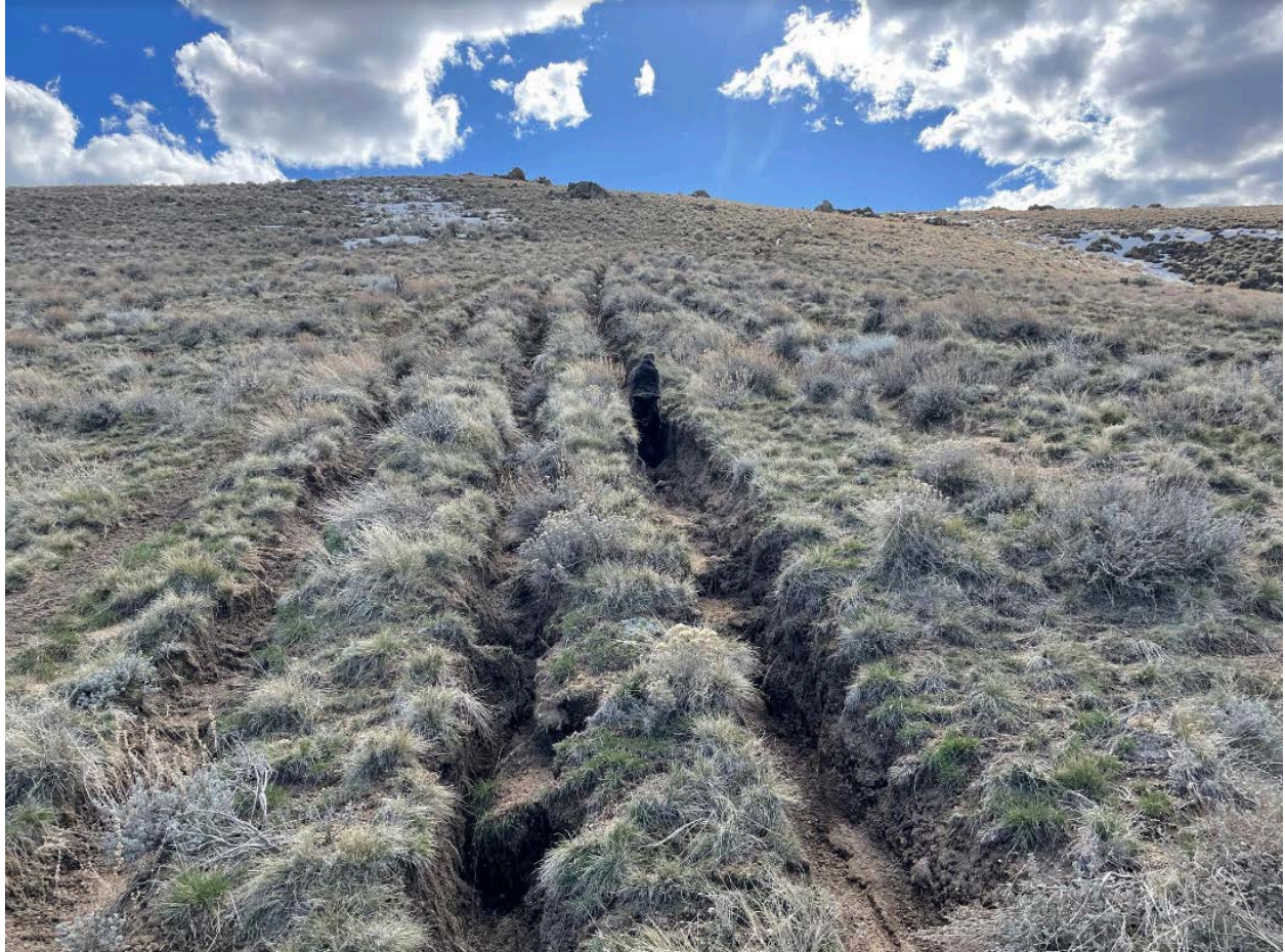
Close up of gully on Gully on 37GV4165.100, south of the junction with Route GVX 1229
