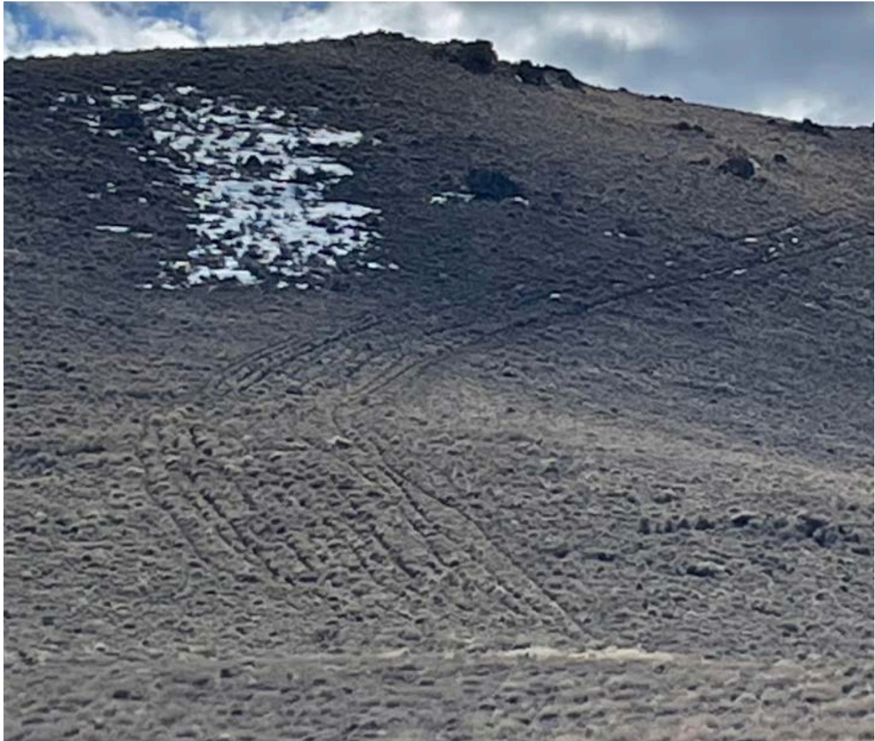
Gullying on 37GV4165.100, south of the junction with Route GVX 1229 from dirt bike tracks
