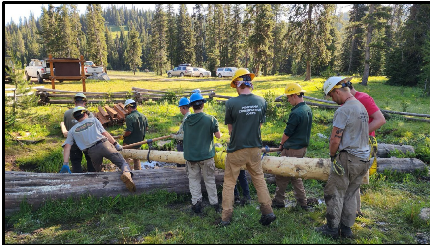
Lifting a stringer into place at the Granite Mountain Bridge
