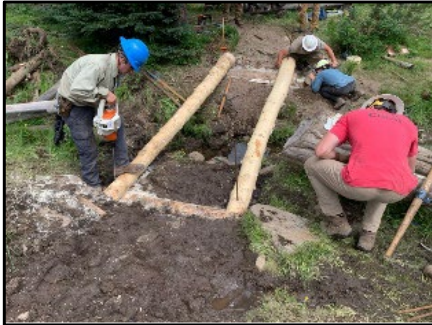
Central Zone Trail Crew and MCC crew members collaborating on the Granite Mountain Bridge stringer installation.
