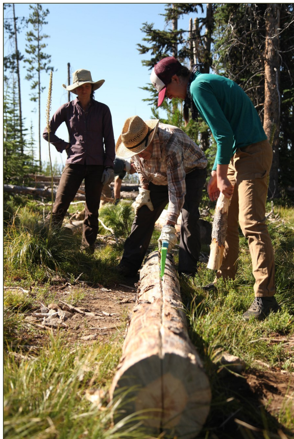
Archaeologists assist volunteer carpenters with splitting a log, which will be used to replace a rotten log segment on the cabin.
