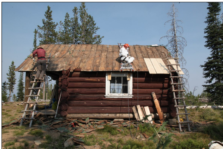
Crews remove old shingles and replace rotten roof sheathing.
