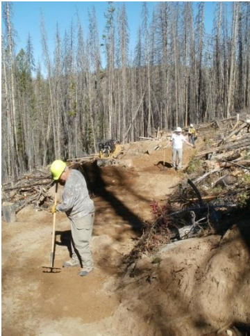
Finish Work on Thunder Mountain
