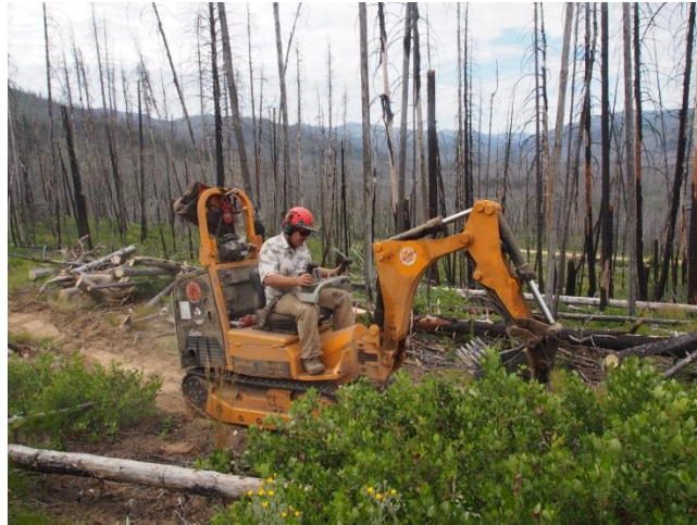
Single Track Machine cutting trail at Wewukiye
