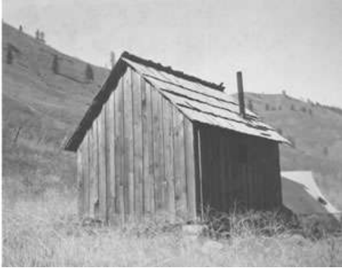
Merle Banks cabin Forest Service photograph
