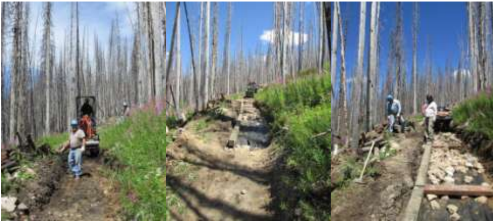
Upper Causeway Construction
