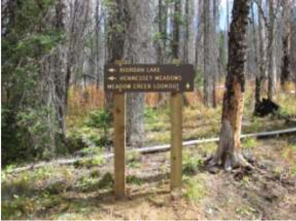
Lower causeway under construction
