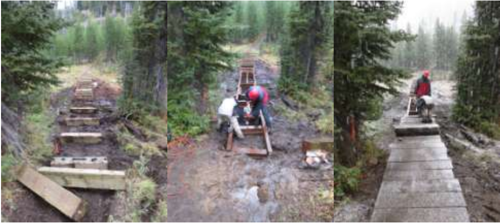
Upper causeway under construction
