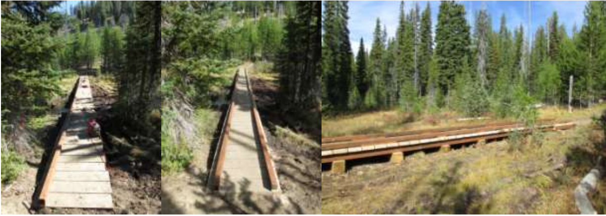
Upper causeway completed
