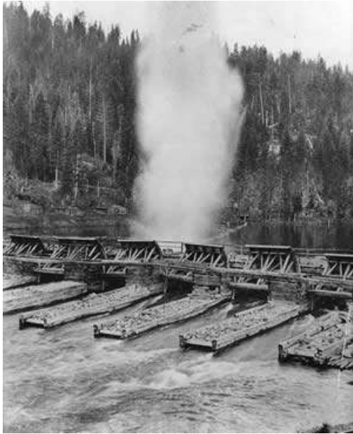
Splash dam on the North Fork of the Payette, below Smith's Ferry
